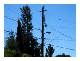
Here is a view of the same utility pole from the side. Note the antennae sticking up from the electric wires to the left of the pole. This device is used to collect usage data from homes and businesses in the area, as part of the 'mesh' network. Usage data from your neighbors can be relayed through your home's smart meter, meaning that there could be far more EMF emissions from your meter than the '45 seconds a day' that PG&E admits to.
