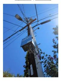
Above is an example of a wireless 'repeater' box that is installed on electrical poles in neighborhoods in advance of PG&E's smart meters arriving.
